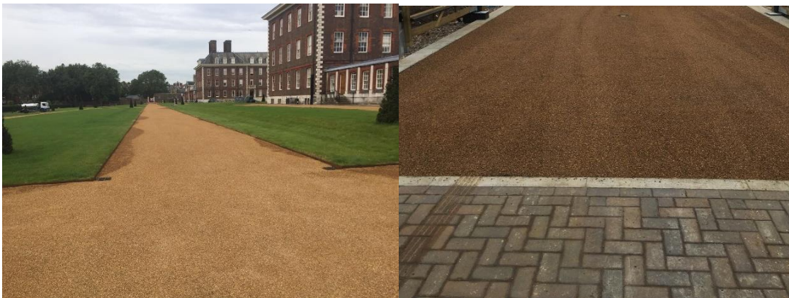
Figure 2: Surface Dressing (Source: Foster Contracting)
